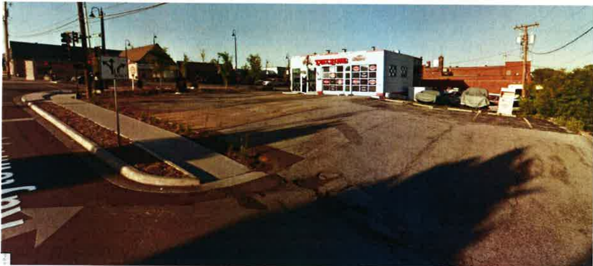
Figure 1 – Street view of proposed Vehicle/Equipment Rental business
